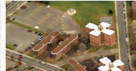
Approved demolition disposition of two Mills low-rise buildings and environmental work on Mills block. This will include site remediation and removal of hazardous building materials where necessary to ensure that new development is free of environmental hazards.
