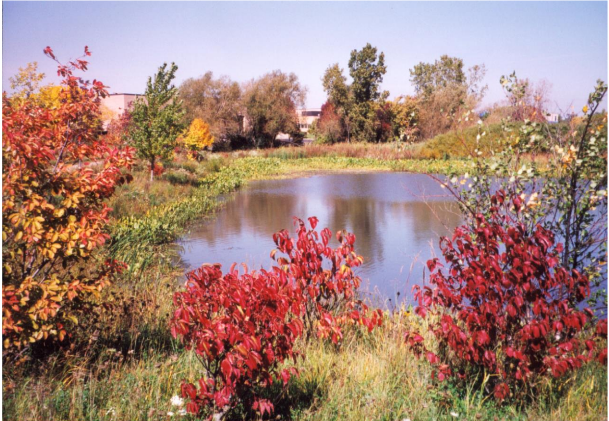
Figure 10, well designed and maintained wetland and stormwater storage area
