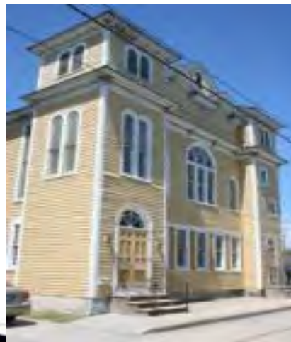
Charles Chipman Cultural Center, Structural Repairs CL Award: $75,000
