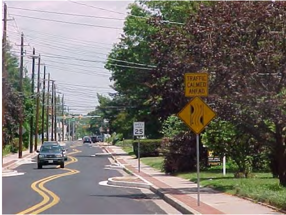
Traffic calming project CL Award: $100,000
