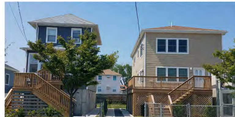
Elevated houses in Queens, New York Photo: NYC Housing Recovery Operations
