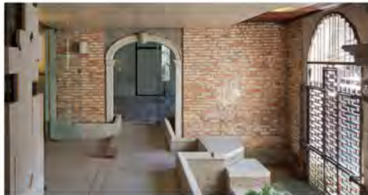
Floodable entryway with stairs that lead to an elevated lobby at the Querini Stampalia in Venice, Italy. Photo: Architects / "The renovation of the Fondazione Querini Stampalia is a great example of how Master Carlo Scarpa integrated the new with the old"
