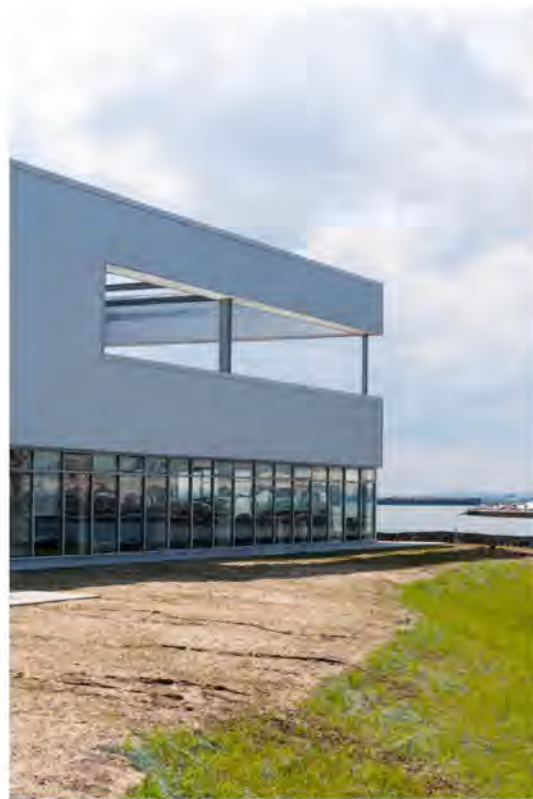
Sunset Park Material Recovery Facility, Brooklyn, New York. Photo by Field Condition / "SIMS Sunset Park Material Recovery Facility"
