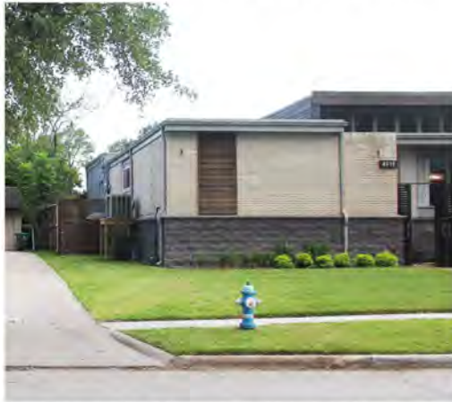
House after elevating. Note that the condenser is also elevated at left. Flood vents are not pictured.
